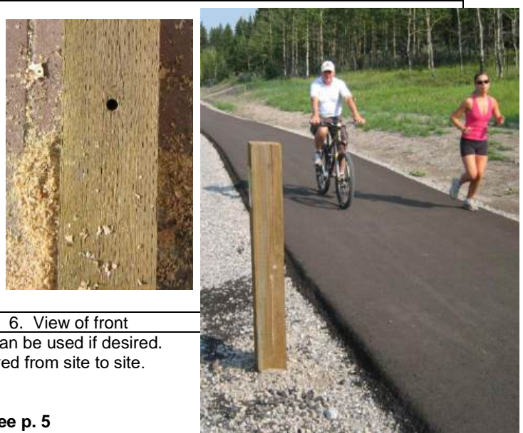
4. Drill hole through post for IR scope; waist height; angle downwards; hole diameter 7/8" for IR scope
