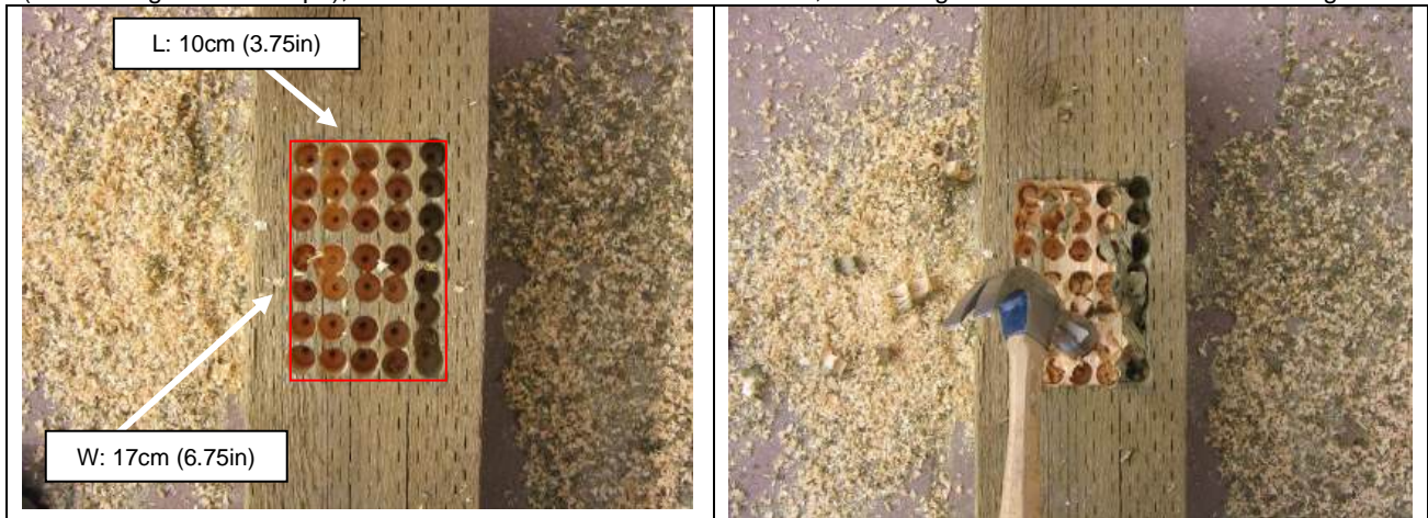
1. Mark chamber area and drill multiple holes to 4.5cm (1.75in) depth; tape drill bit to mark depth
