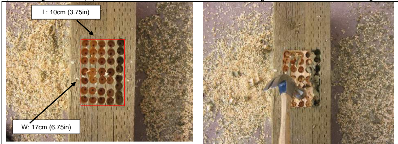
1. Mark chamber area and drill multiple holes to 4.5cm (1.75in) depth; tape drill bit to mark depth
