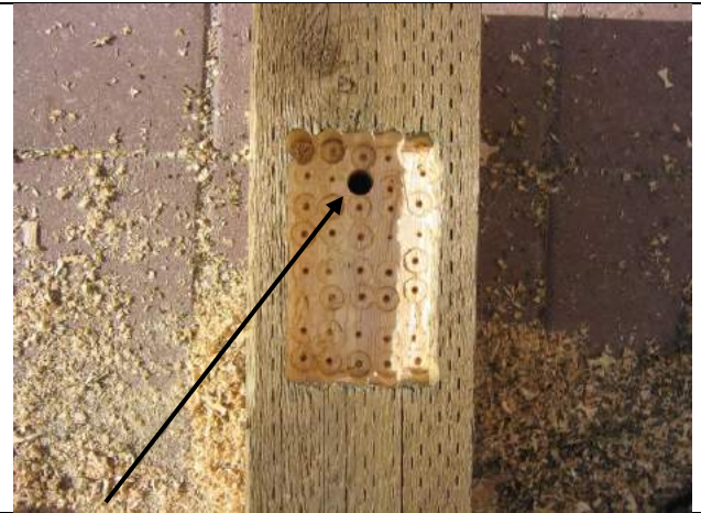
4. Drill hole through post for IR scope; waist height; angle downwards; hole diameter 7/8" for IR scope
