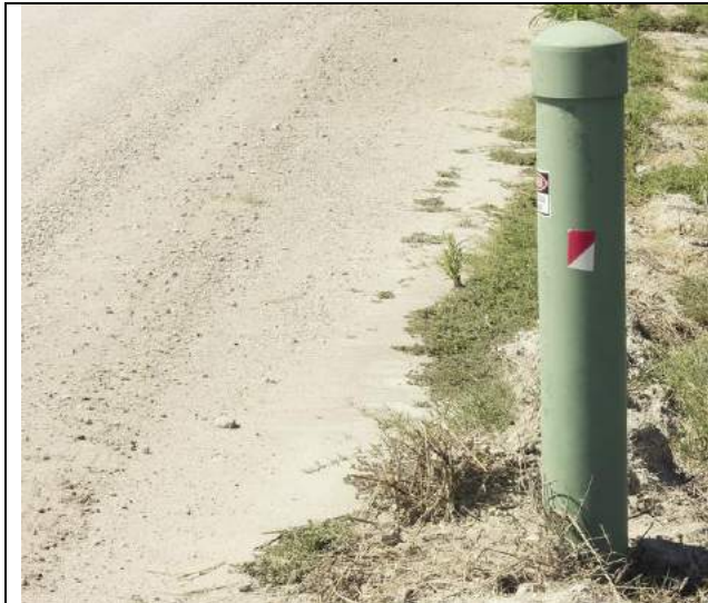
PVC Post Installation
