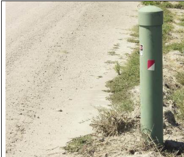
PVC Post Installation
